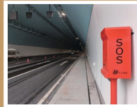
Highway tunnel in Chongqing, Gaoteng
